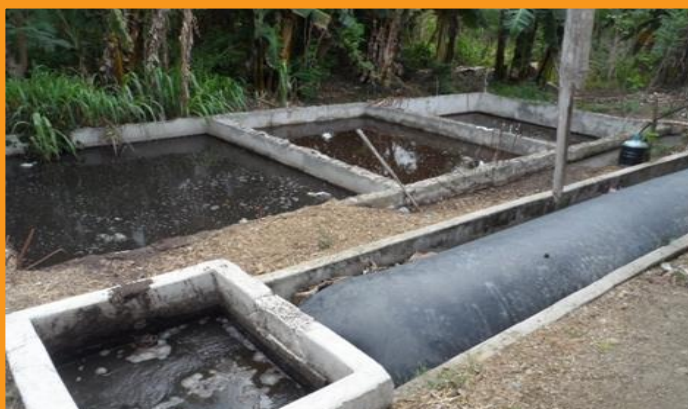
Mixing Pit (top) and Tube Digester (bottom)
